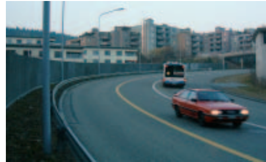
Fig. 2: Road traffic noise situation showing barriers and reflective elements that can be handled by the new calculation model.
