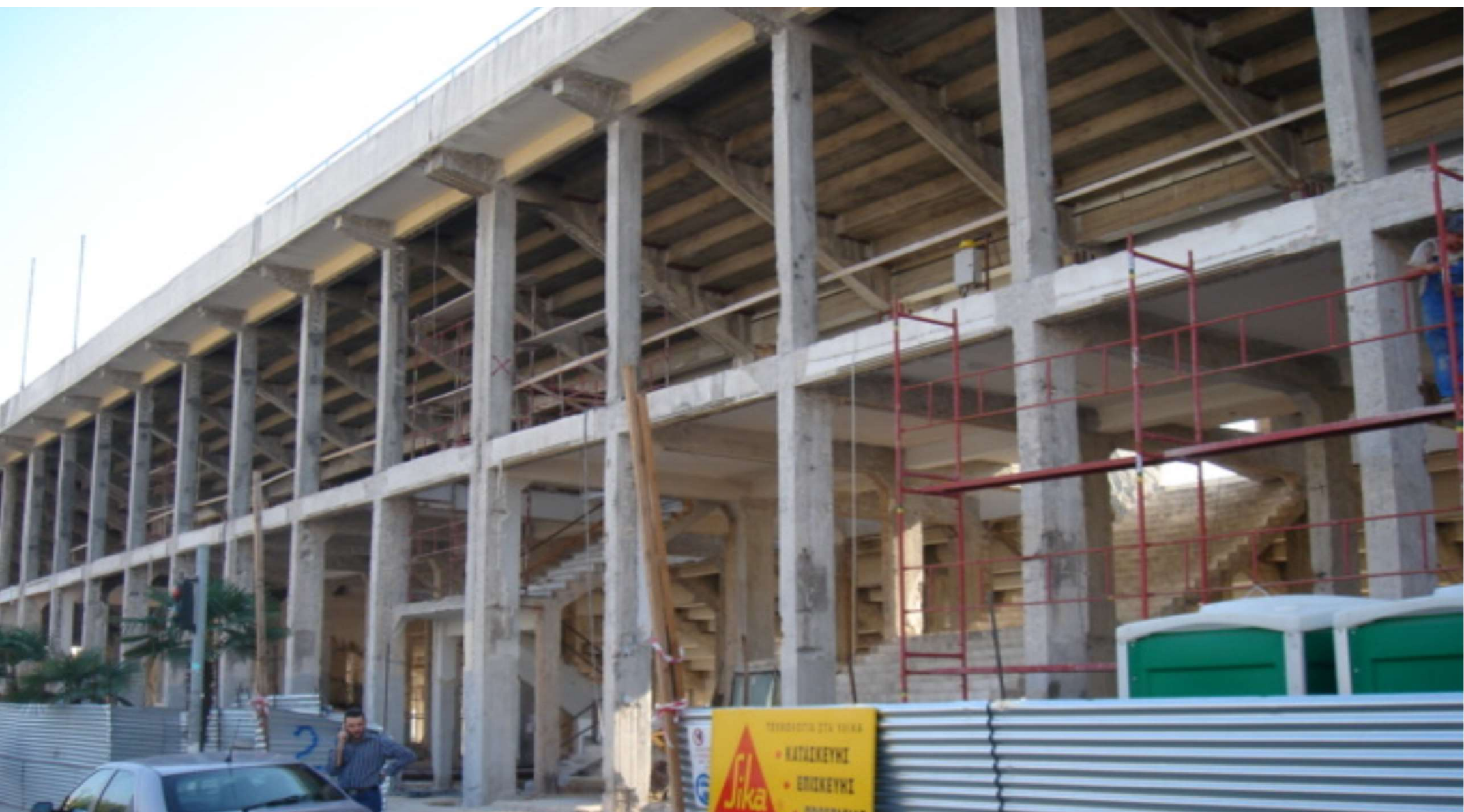
Seismic retrofitting of column-beam joints of Aigaleo football stadium in Athens, Greece, using CFRP fabrics with steel anchorages
