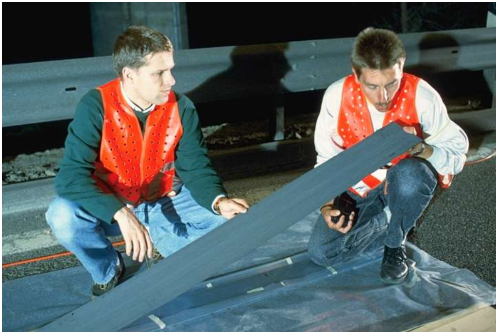
Externally Bonded FRP: Flexural
