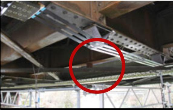
The PUR system now provides bridge operators with a swift, cost-effective alternative to bridge replacements. Wear and tear can be reduced to such an extent that, in theory, fatigue can be deferred indefinitely. While project head Masoud Motavalli is more realistic when it comes to practice, he remains confident: “A bridge reinforced entirely using this method will certainly last for the next 50 years, by which time we’re bound to have devised new methods to repair ageing bridges.”
