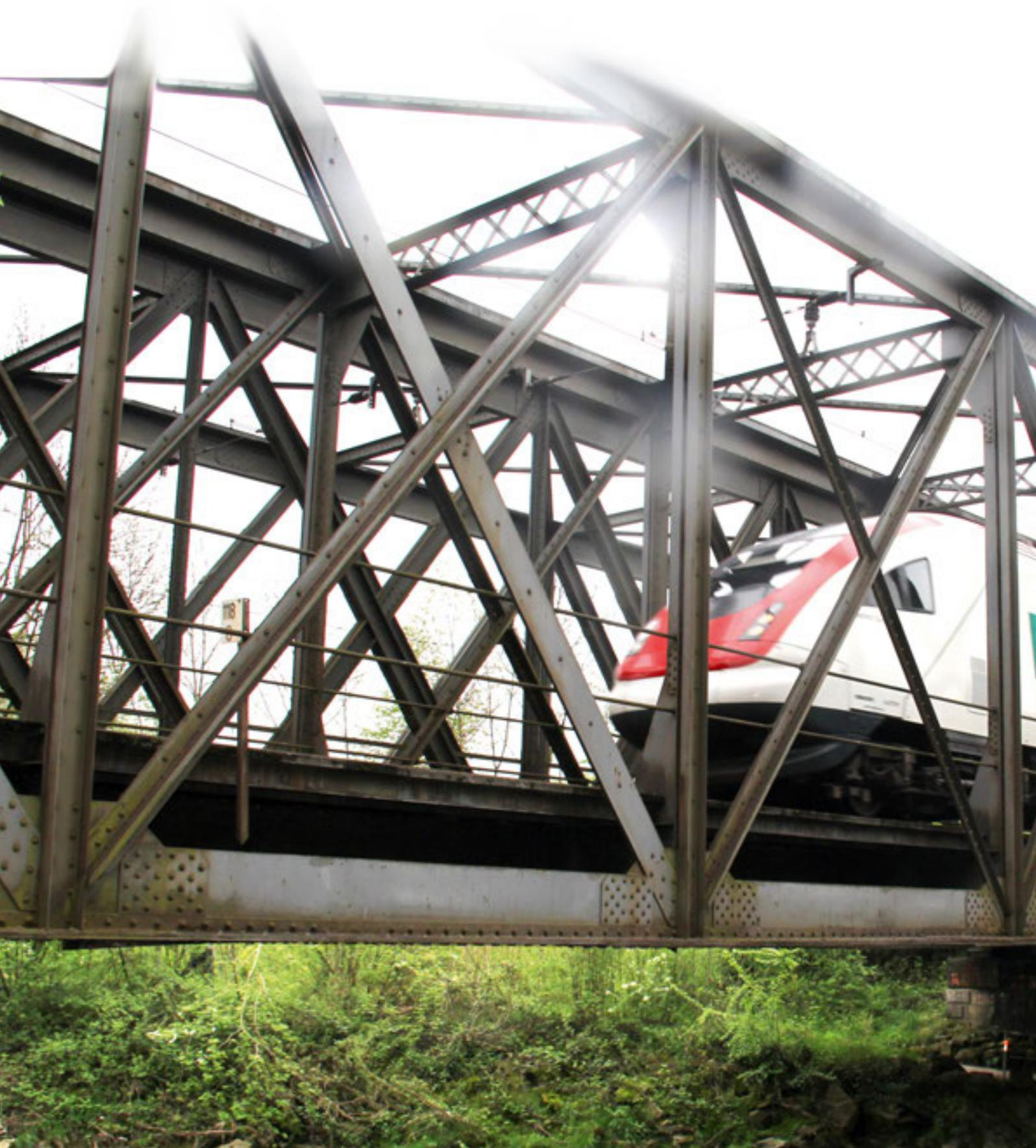
An increasing number of steel bridges need to be replaced or repaired due to signs of fatigue. Researchers from Empa fortify the load-bearing elements with pre-stressed, fiber-reinforced plastic plates – a cost-effective alternative to building a new bridge. The recently patented method was now used on the 120-year-old Münchenstein Bridge.
