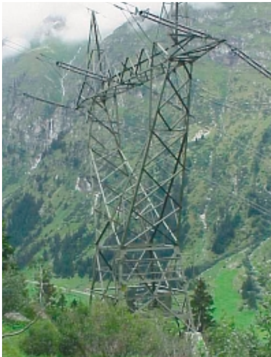
Fig. 1: Pylon of power transmission line with optical fibers inside the ground wires.
