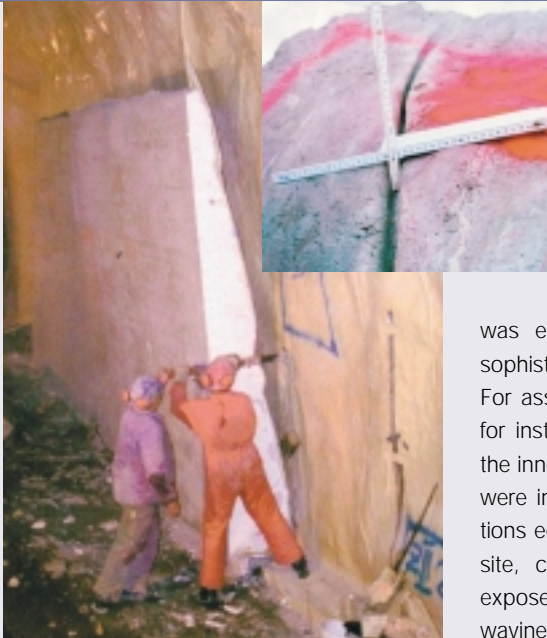
Removal of the concrete support shell for the inspection of the waterproofing membrane.
