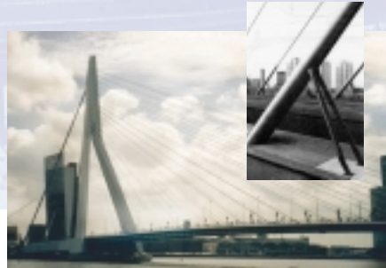
A typical example of a cable-stayed bridge: the Erasmus bridge in Rotterdam. The inset shows the passive viscous dampers, which were installed to reduce cable resonance.
