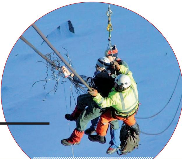
Crack in the cable of the Schilthornbahn cable car
