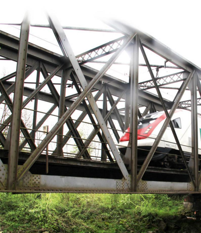
An increasing number of steel bridges need to be replaced or repaired due to signs of fatigue. Researchers from Empa fortify the load-bearing elements with pre-stressed, fiber-reinforced plastic plates – a cost-effective alternative to building a new bridge. The recently patented method was now used on the 120-year-old Münchenstein Bridge.
