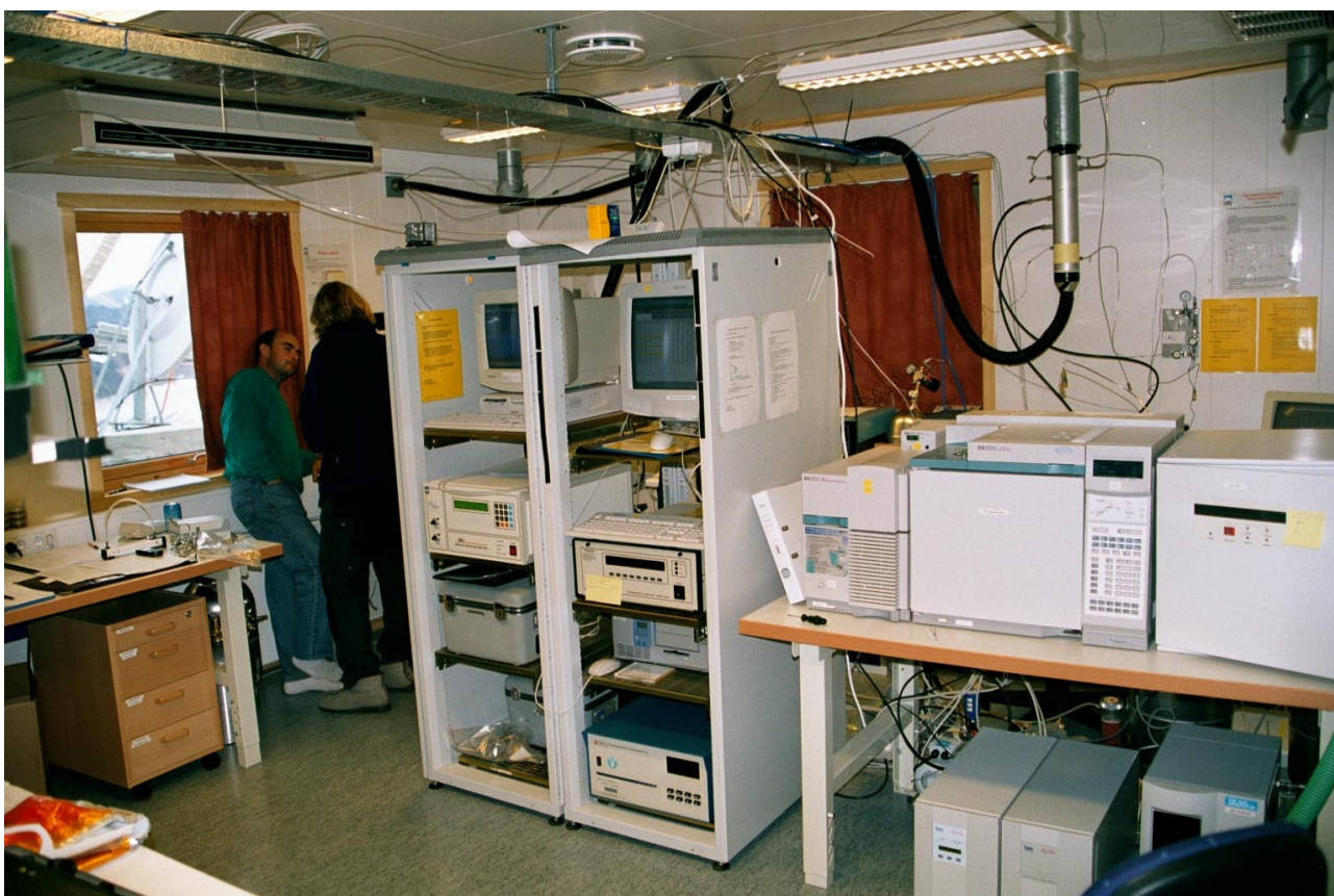
Figure 6: Inside the new laboratory at the Zeppelin Station
