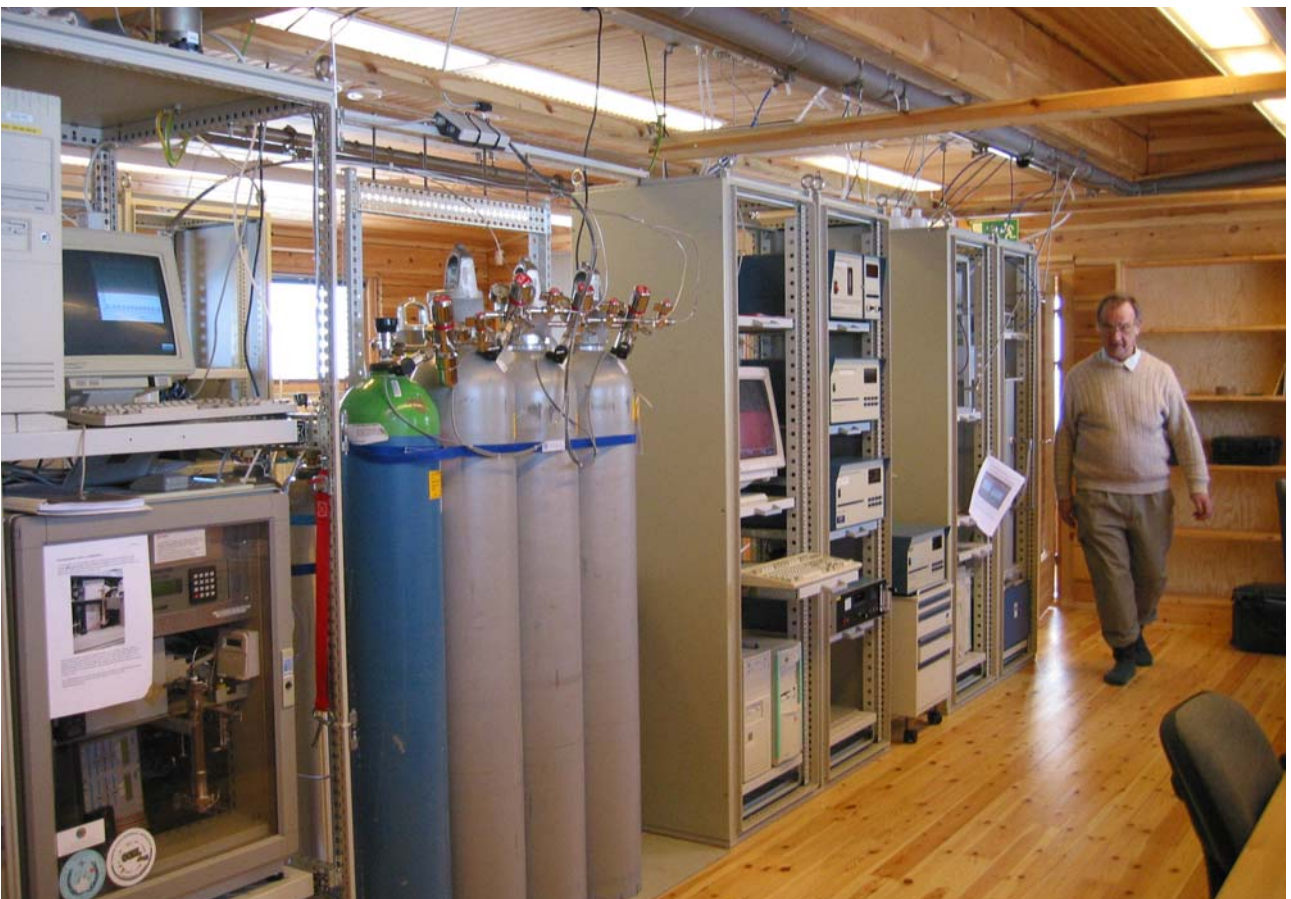
Figure 5: Inside the laboratory building at the Pallas Sammaltunturi GAW station
