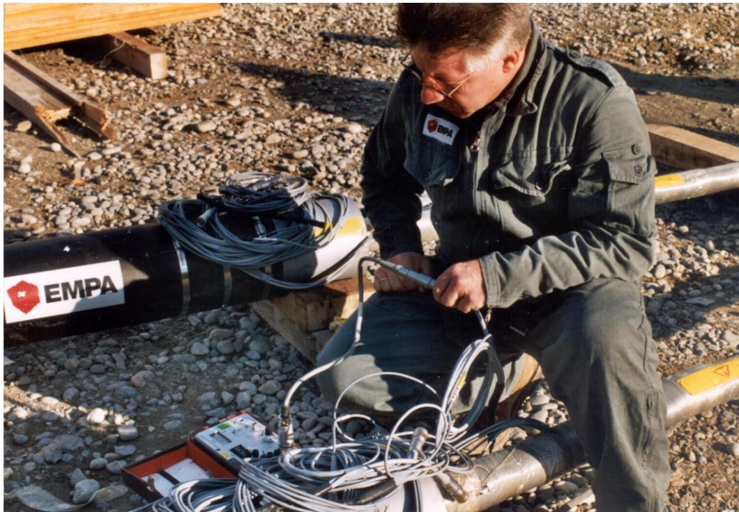
Fig.2: Testing an RSG wiring on a stay cable made of carbon reinforced polymer (CFRP).
