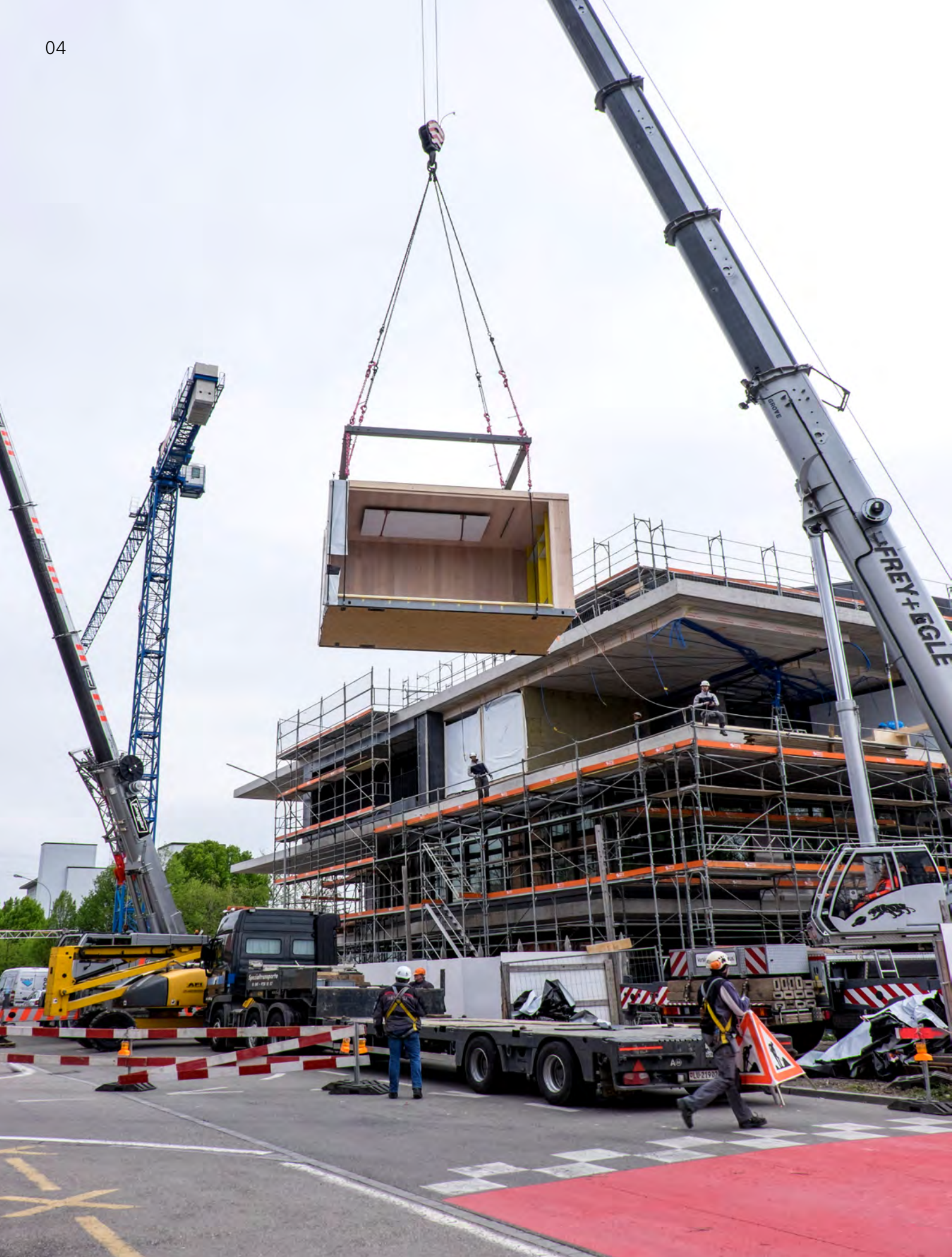
Installation of the prefabricated modules for the unit Vision Wood on April 26, 2016.
