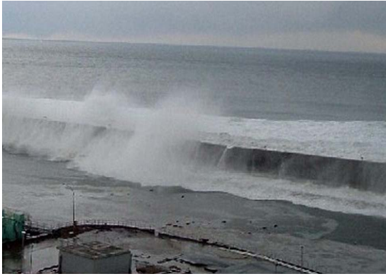
Figure 8: Sea wall breach.
