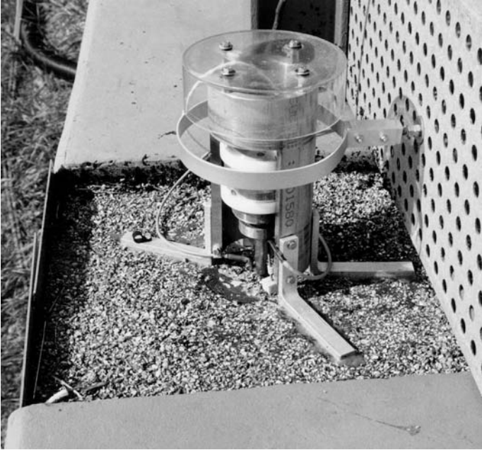
Figure 5. In situ set up on the bridge asphaltic plug joint consisting of rheometer with protection shell, lateral support, temperature and light sensors
