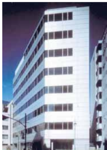
The aluminium façade of the YKK building in Sendai, Japan, is coated with titanium dioxide, which makes it practically self-cleaning.
